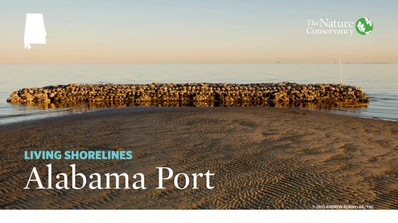
Alabama Port is located just south of Mobile County's Bayfront Park and runs parallel to the Dauphin Island Causeway. The shoreline has been experiencing significant erosion since the 1950's. Reef segments were placed about 100 ft waterward from the shoreline and fronted more than 4,471 ft of natural shoreline. The project restored almost 1 acre of reef breakwater and living shoreline habitat.
